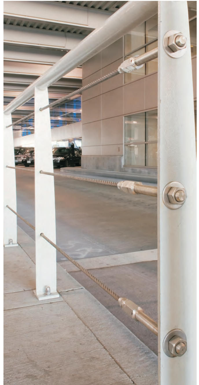
Stud Fitting - Pedestrian Walkway - Portland International Airport
