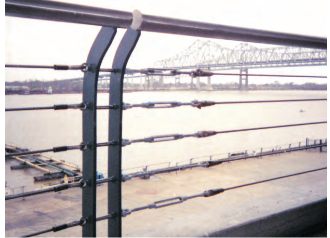
Open Body Turnbuckles - Riverwalk Railings - New Orleans, LA
