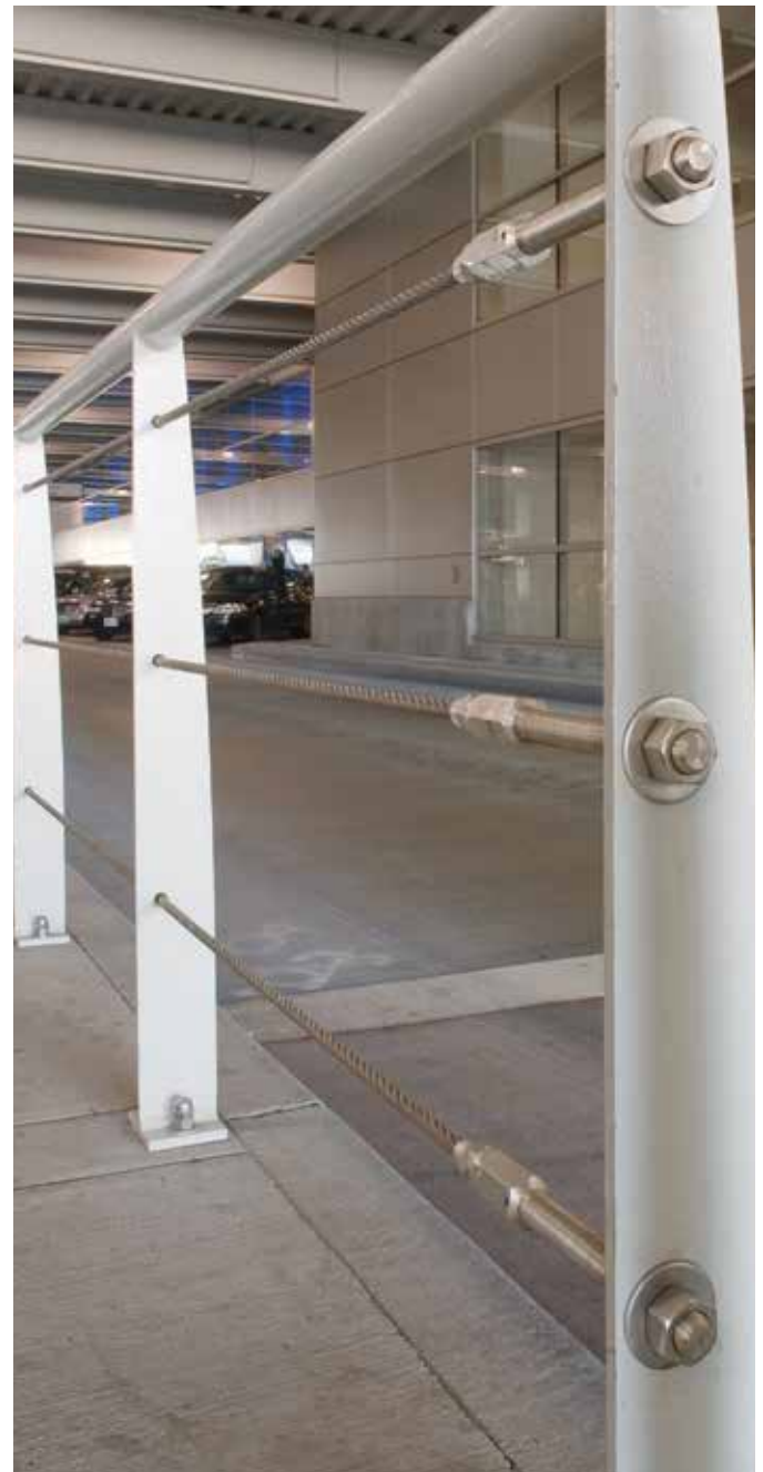
Stud Fitting - Pedestrian Walkway - Portland International Airport
