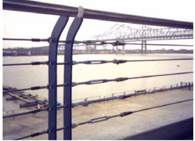
Open Body Turnbuckles - Riverwalk Railings - New Orleans, LA
